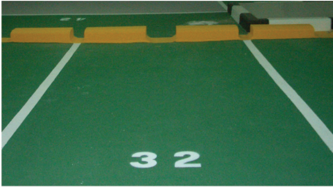
NATIONAL GUARD EPOXY FLOORING TOPCOAT
